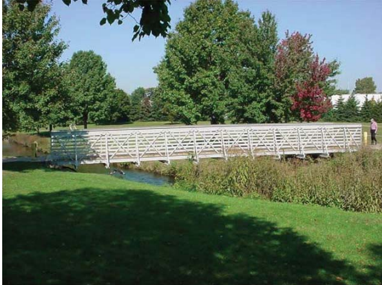
Figure 3 All fiber reinforced polymer pedestrian bridge.
