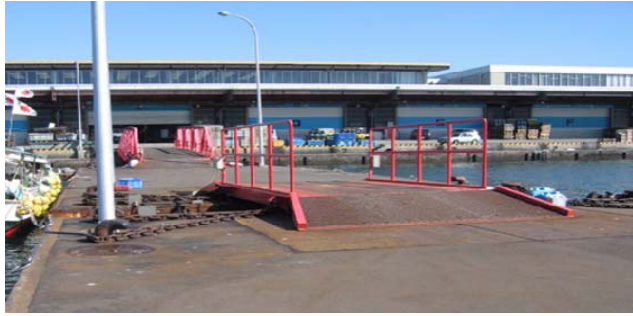
Figure 2: A pier footbridge
