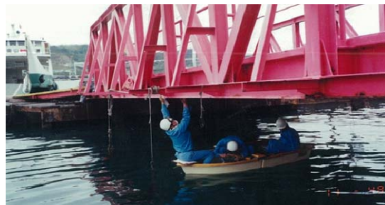
Figure 5: Inspection of a pier bridge
