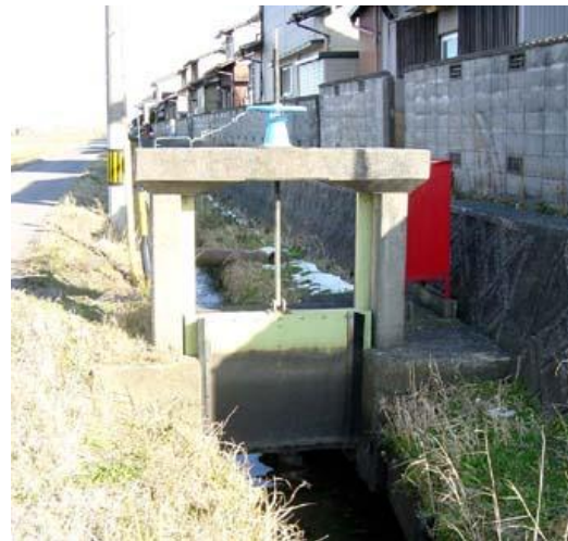
Figure 4: FRP gate in use for 35 years
