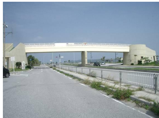
Figure 1: Okinawa Road Park Bridge (The first all FRP pedestrian bridge in Japan, Okinawa Prefecture, 2000)
