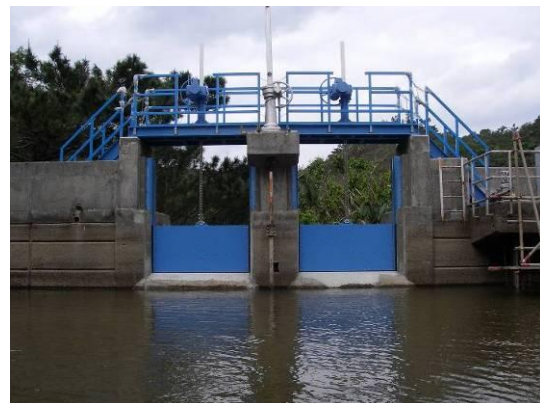
Figure 3: FRP gates at Komagari dam (Ogasawara, 2007)
